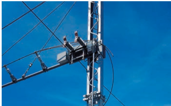
Single-pole or two-pole, earthing switchgear in withdrawable execution Single-pole or two-pole, earthings switch for assembling on pole or wall
